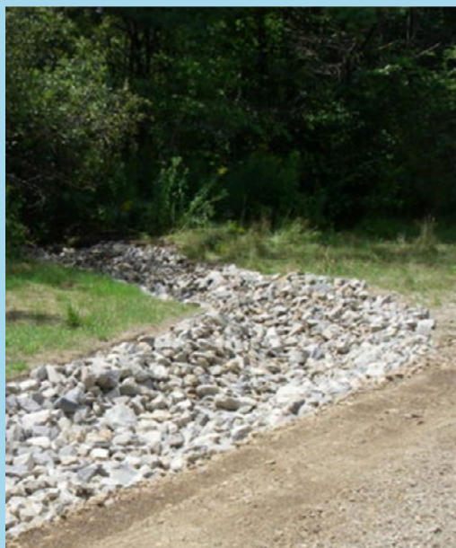
Riprap lined ditch turnout into existing vegetation.
