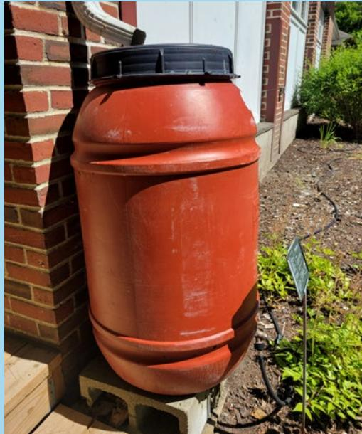
A single rain barrel with a drip hose connected to the spigot.
