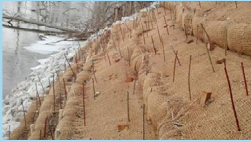
Slope stabilization using live stakes of dogwood & willow with coir blanket and slope interruption to control temporary erosion.
