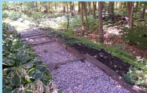
Retrofit existing steps by excavating behind each step and adding crushed stone.
