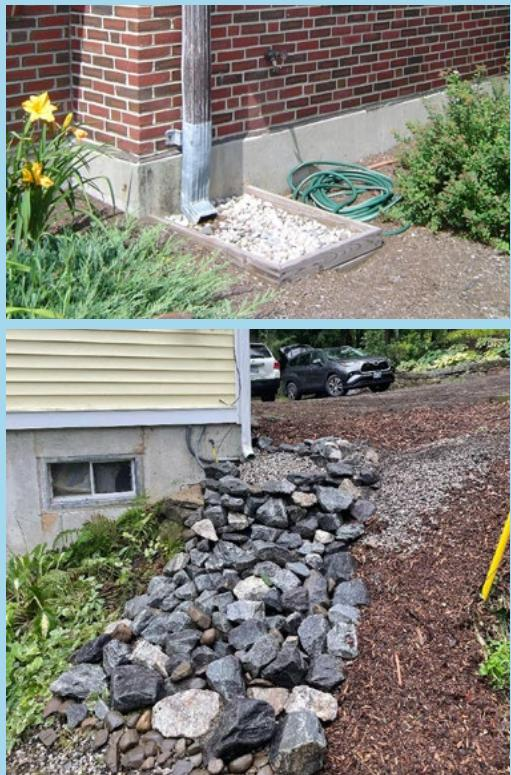
Drywells should be placed in areas that receive concentrated flow of runoff such as below gutter downspouts. A stabilized outlet can be constructed to handle overflow (bottom image).
