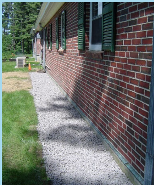
A fully installed dripline trench along a section of building with no gutters.
