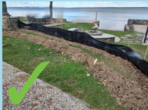
The silt fence on this site is entrenched properly with space to pond water for sedimentation to occur.
