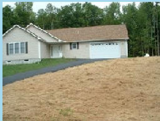
A thick coat of hay mulch is a great way to temporarily stabilize bare soil. The ground should not be visible through the hay.
