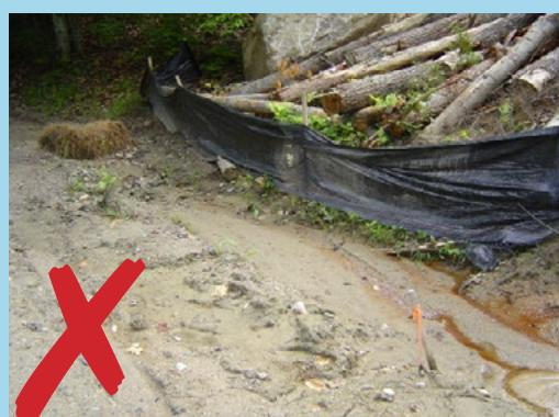
The silt fence on this site is NOT entrenched so sediment is easily able to leave the site unchecked.
