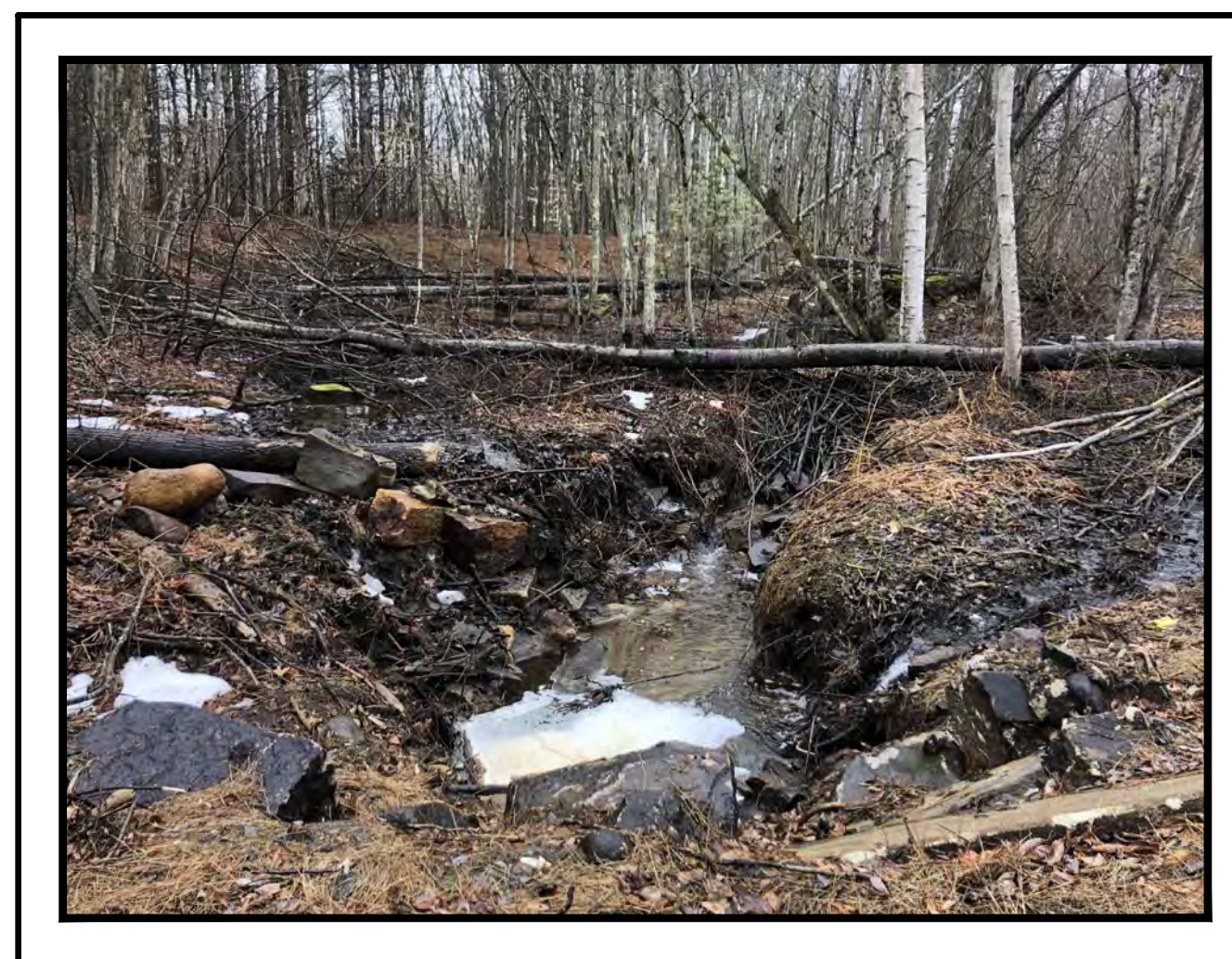
GRANITE CULVERT AT INLET (LOOKING UPSTREAM) NOT TO SCALE
