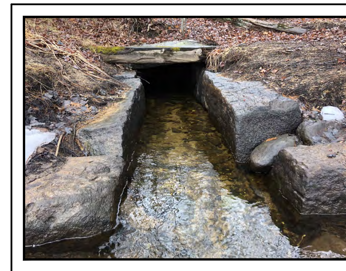
GRANITE CULVERT AT OUTLET (LOOKING UPSTREAM) NOT TO SCALE
