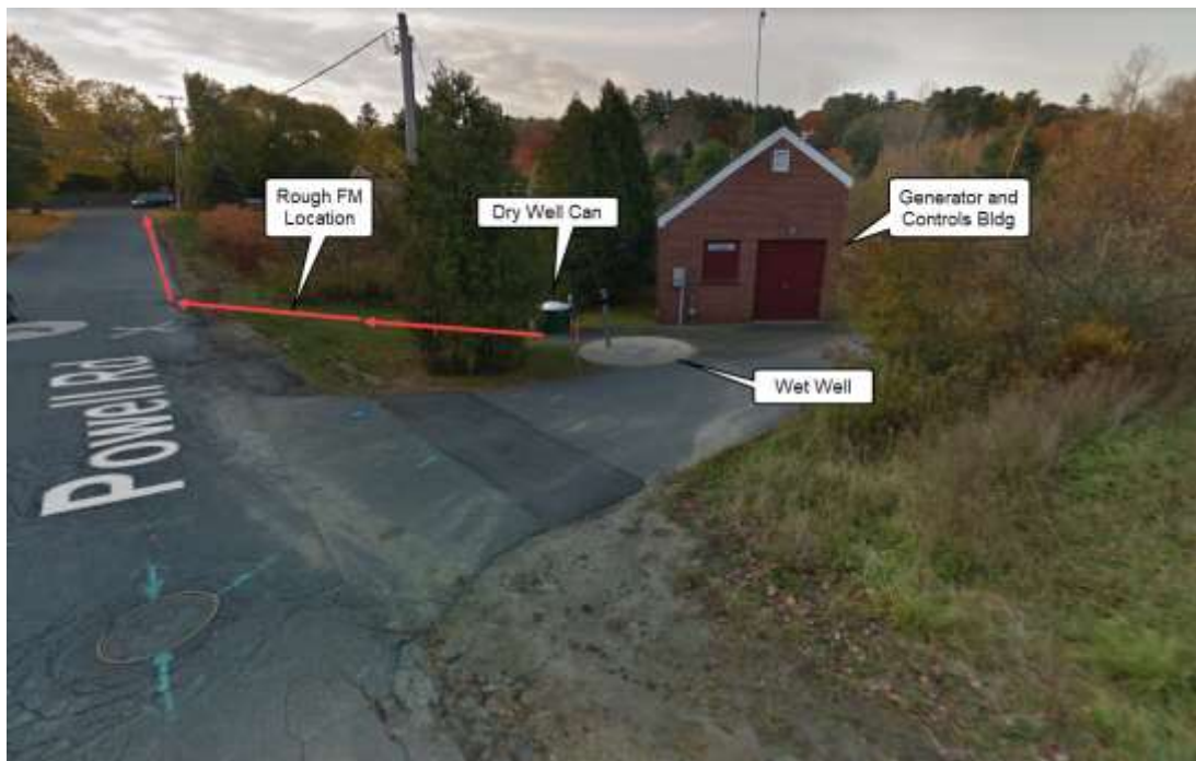
Figure 1: Powell Rd. Pump Station, Street View
