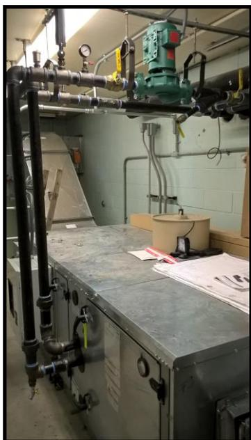
**Headworks HVAC Upgrade** – 2018 CIP 424, project 2571 - Main air handler and hydronic piping during construction. The system was brought online Summer 2021.
