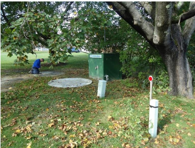
**2016 – Longmeadow P.S.** installed in 1983 – condition rating was 3.26 - Upgrades included new SCADA and pump control panels, pumps, valves, and electrical work. New rating is 4.56
