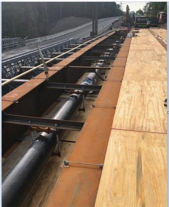
**2020 CIP 60, 43 Project #3212** Little River Bridge Replacement – Force Main and Water Main replacement in conjunction with the MDOT replacement of the bridge
