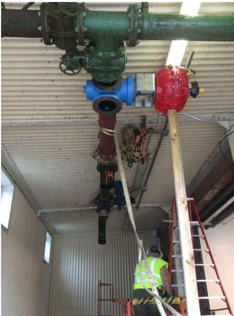
**2019 CIP 416 project 3001 - Cake Unloading Valve during installation**
