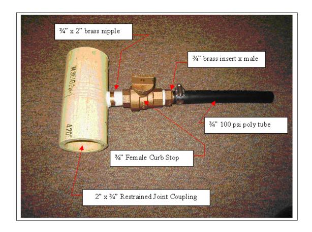
Temporary service line boiler drain assembly used for customer garden hose connection.
