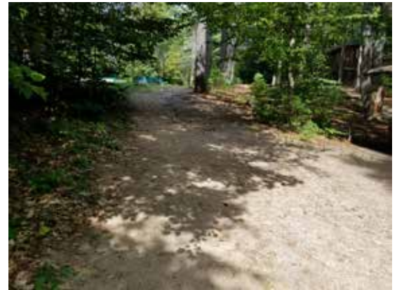
Before – eroding hillside
