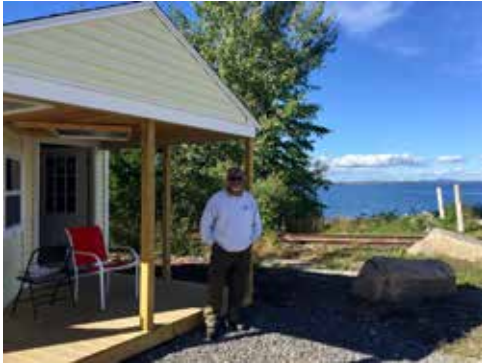
The District's new boat launch shelter
