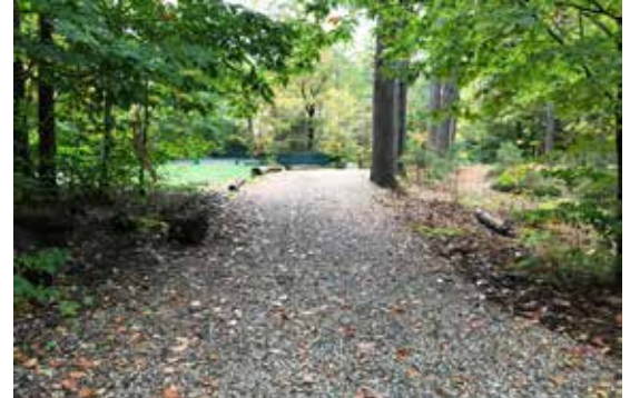
After – hillside stabilized with Geoweb filled with crushed stone
