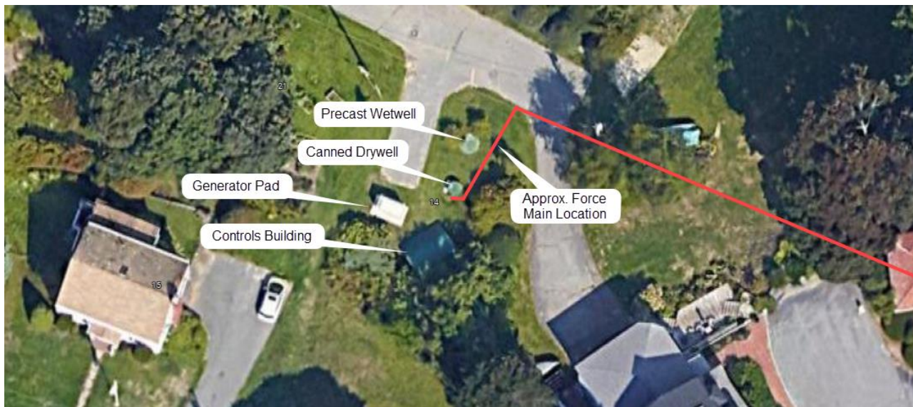
Figure 1: Ottawa Rd. Pump Station, Aerial View
