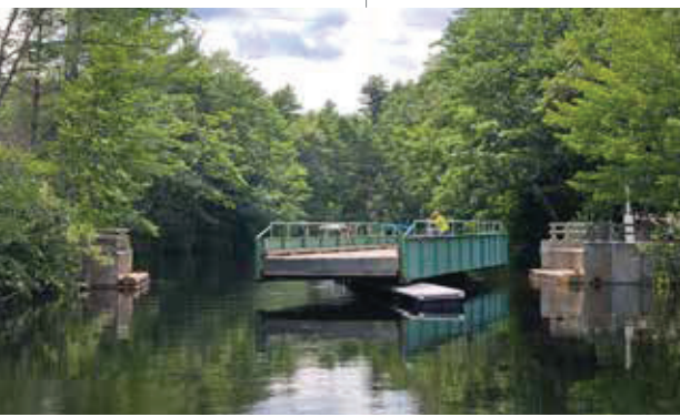
Songo Lock, constructed in 1830, is the last surviving lock of the Cumberland and Oxford Canal, a 19th-century canal in southern Maine. The lock is located on the Songo River, just above its confluence with the Crooked River at the northern end of Sebago Lake State Park in the town of Naples. It allows boats to navigate between Long Pond and Brandy Pond at higher elevation to Sebago Lake at lower elevation.
