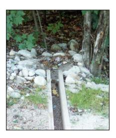
Install the culvert flush with the surface of the road. If placed too high, stormwater will not enter the structure; if placed too low, it may quickly fill with road material and sediment loosened during installation.
