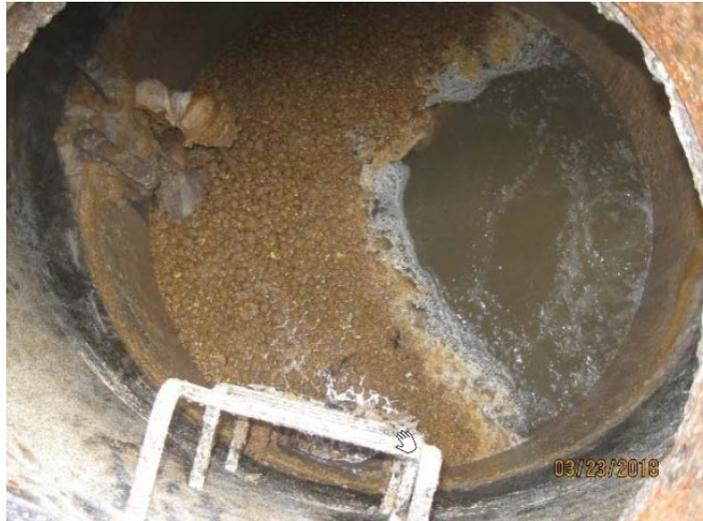
*Photo caption: grease build up in a pump station is one example of a sewer system problem.*
