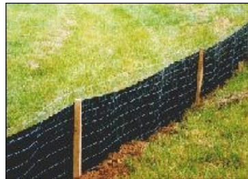
Properly installed silt fence, buried at the base.
