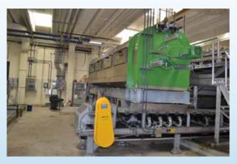
SOLIDS HANDLING: A 2018 replacement of the Westbrook/Gorham/Windham Regional Wastewater Treatment Plant's dewatering system has reduced the cost and volume of biosolids that are disposed from the treatment plant. Significant investment in the East End Wastewater Treatment Plant's solids management systems were made to keep the systems operating efficiently.
