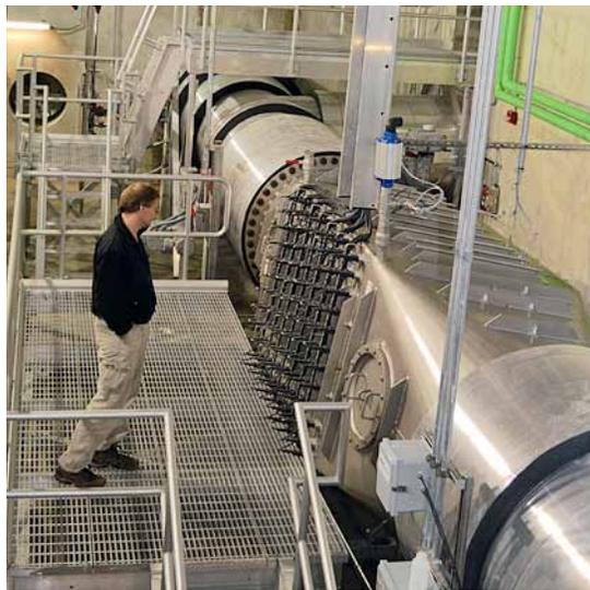
Two-14-ft., 84-lamp UV units are installed in an underground chamber. Each UV unit connects to a 48-inch pipe and has the capacity to treat the Plant's full capacity of 52 MGD.
