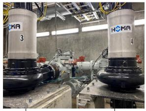
Dana Court Pump Station New dry pit submersible pumps installed in 2019
