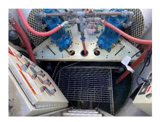
**Garrison Street Pump Station - Controls / Pneumatics Pumps**-2021 CIP project #3184 under design to replace ejector style pump station with submersible pump station
