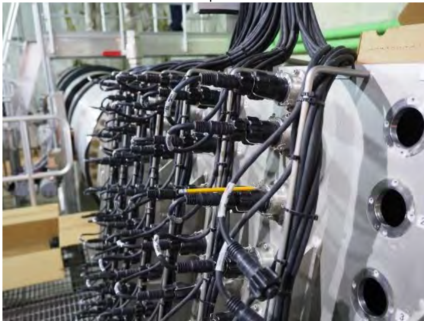
UV Reactor #1 Lamp Power Connections
