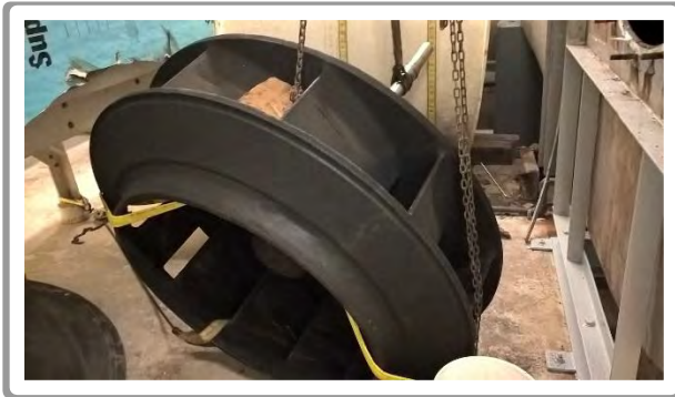
Completed EEWTF Odor Control rehabilitation including 45,000 cfm fan.
