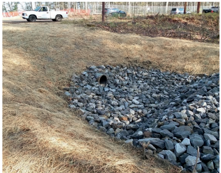
Level lip spreader installed to prevent ditch erosion
