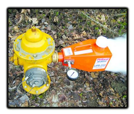
In an effort to improve the water quality in the distribution system, the District performs multi-directional flushing to remove any sediment that deposits on the bottom of these mains. This sediment can cause a reduction in the area's chlorine residual and increase customer's water quality inquiries.
