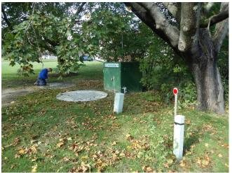
2016 – Longmeadow P.S. installed in 1983 – condition rating was 3.26 -Upgrades included new SCADA and pump control panels, pumps, valves, and electrical work. New rating is 4.5
