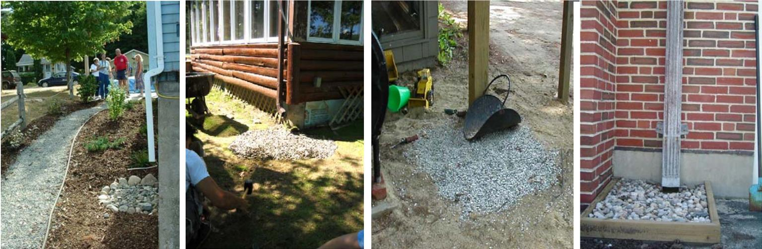
**Purpose:** Drywells collect and infiltrate runoff at gutter downspouts and other places where large quantities of concentrated water flow off rooftops. These systems help control erosive runoff on your property, and reduce wear on your house by minimizing back splash.
