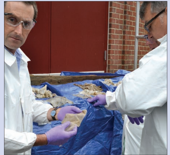
Representatives from the consumer wipes industry study the material collected from the $2.5 million screening system that was installed at the Cottage Place Pump Station in Westbrook to remove wipes that are flushed into the wastewater system.
